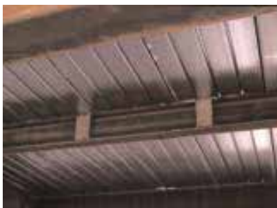
Noggings glued between steelwork flanges
