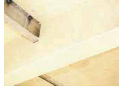
CONLIT® 150 T With a white glass tissue factory-applied to the outer face.
