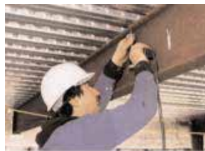
Fixing stud welded pins
