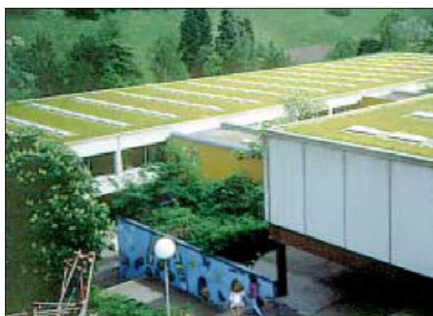
Extensive roof garden
